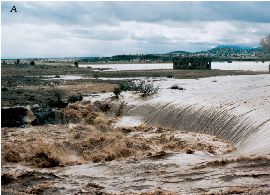
Figure A13. Photographs showing A, flood of February 20, 1993, at Sullivan Lake dam. View to southwest. Sullivan Lake dam is behind hydraulic drop. B, Verde River gorge below the dam. View downstream to east. Canyon is carved from Tertiary basalt. Peak discharge of 23,200 ft 3 /s and daily mean discharge of 13,700 ft 3 /s are the sum of Big Chino Wash, Williamson Valley Wash, Little Chino Creek, and Granite Creek at Paulden gauge. Photographs by E. Carr.
