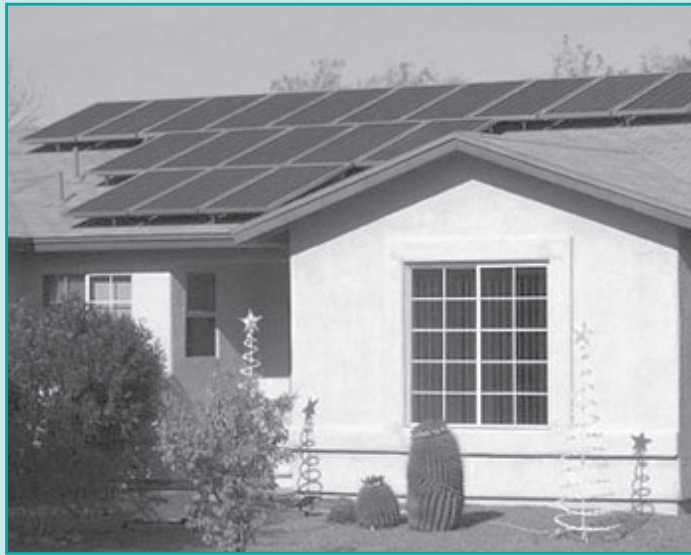
This solar-powered home in Tucson, Arizona makes energy out of the region's abundant sunshine. Source: GeoInnovation.
