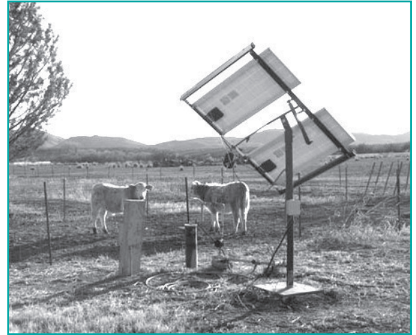
In rural Arizona, solar panels are commonly used to provide power to water supply wells where electric utilities are not available. Source: Richard Conway.
