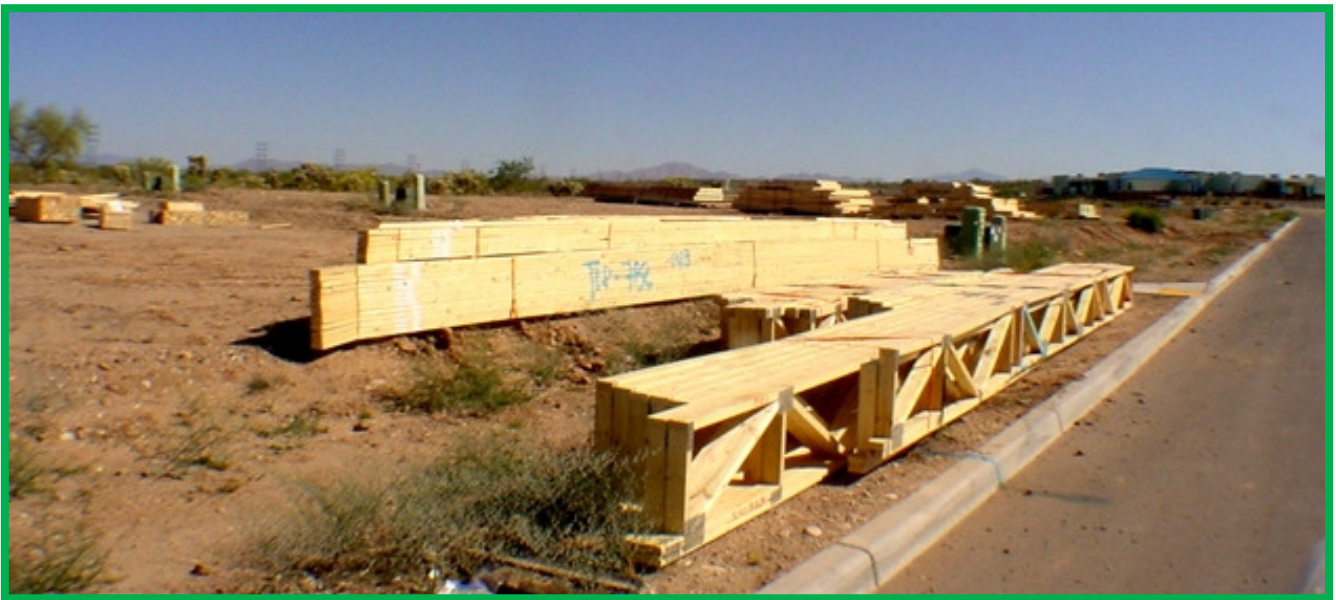
Photo 1 - Sierra Morado, Phase II Construction
