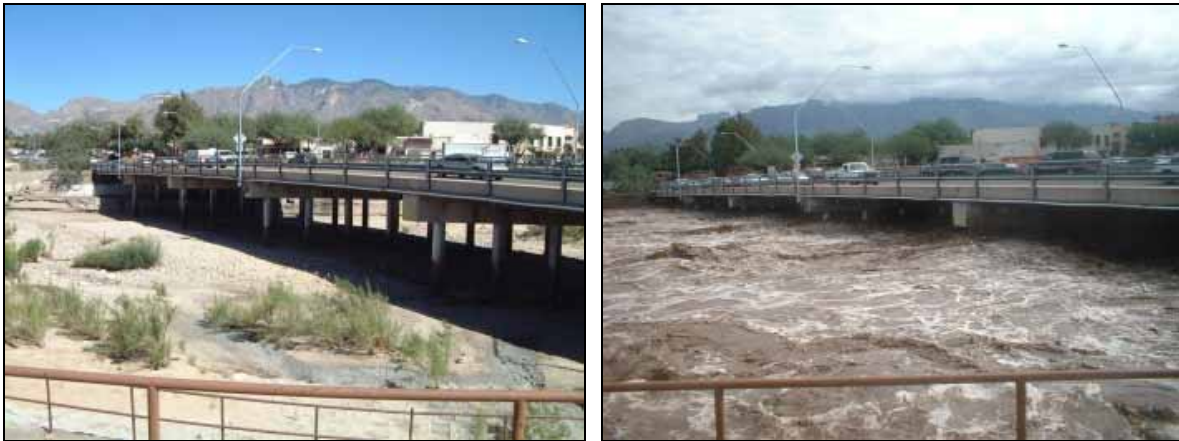
Figure 39. Photographs of the Rillito River, Tucson, Arizona, dry (left) and with flow (right).
