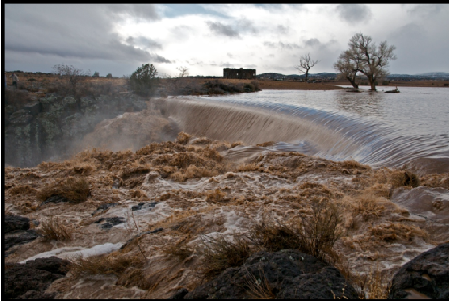
Figure 6. Winter storm flood flow overtopping Sullivan Dam (January 21, 2010). Photo credit: Gary Beverly
