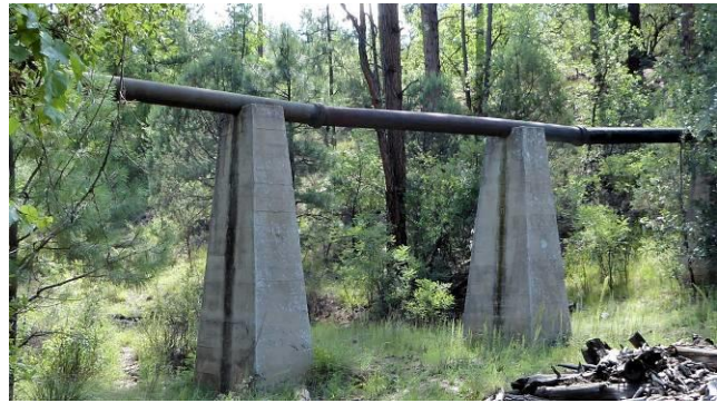
Old pipeline from Goldwater Lake to Prescott
