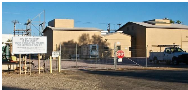
Water production facility in Chino Valley Gary Beverly photo
