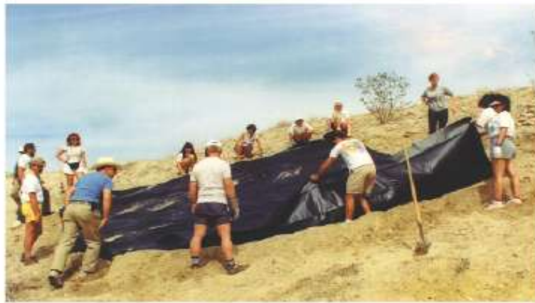
Placing the catchment liner
