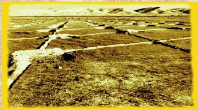
Microcatchment construction — Israel
