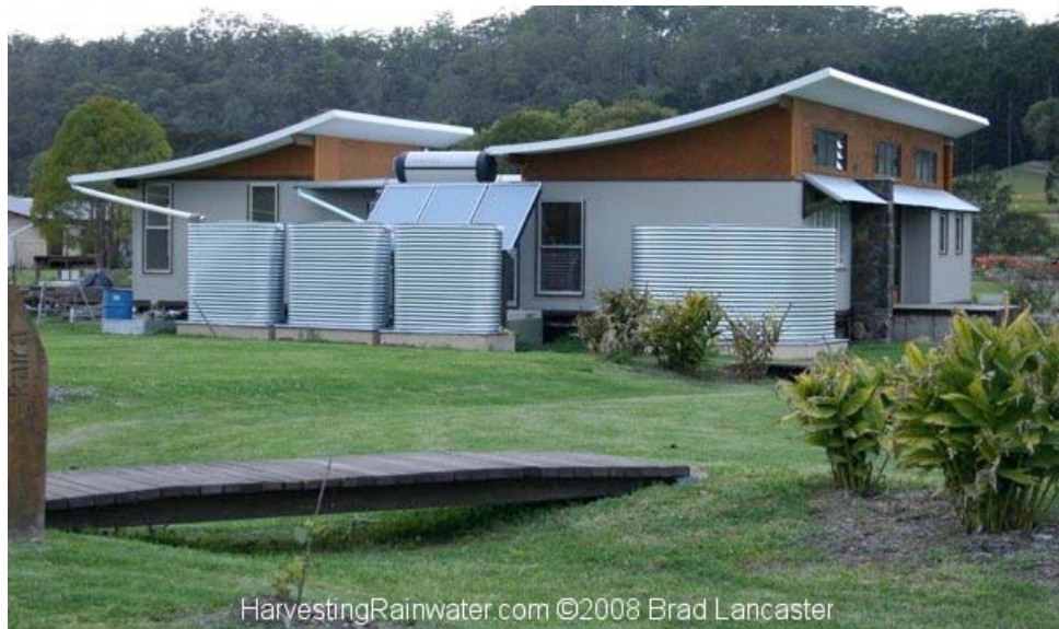
Figure 4: Cisterns harvesting roof water (Lancaster 2008).
