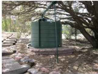
Installed by AZ Seamless Gutters
