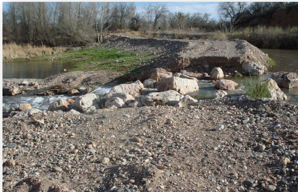
Figure 6.10. Cottonwood ditch diversion dam on the Verde River, breached, presumably by a winter flood event. Photo taken March 15, 2007. Courtesy of Jeanmarie Haney, The Nature Conservancy.
