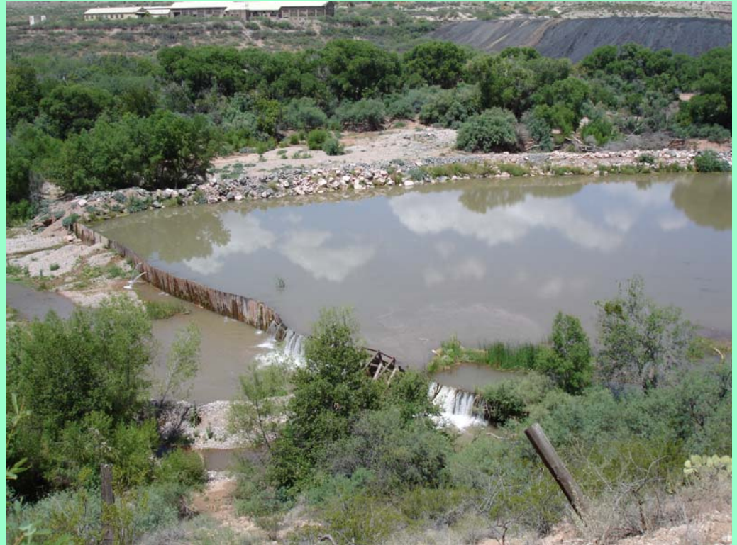
Brewer's Tunnel Diversion
