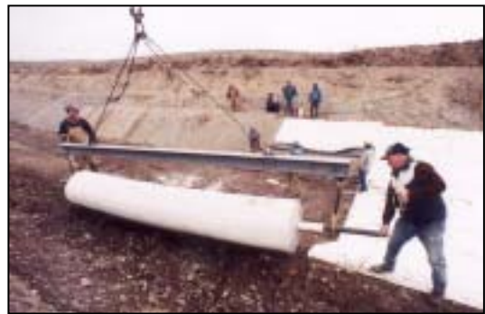
Installing canal lining technologies
