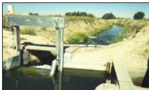
Modernized Canal Structure
