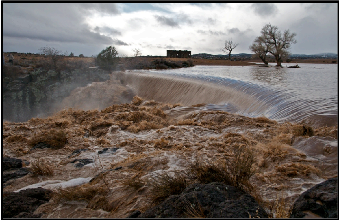
Photo 69. Winter storm powers 5000 cfs flood flow overtopping Sullivan Dam, just upstream of the study area boundary.
