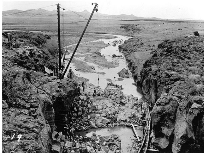
Figure 2.15 —Photo from 1937 showing the building of the Sullivan Dam wall. Note the scarcity of woody plants and the additional seasonal flow—probably runoff from Big Chino Wash and baseflow from Del Rio Springs. (Photo courtesy of the Sharlot Hall Museum, Prescott, Arizona.)
