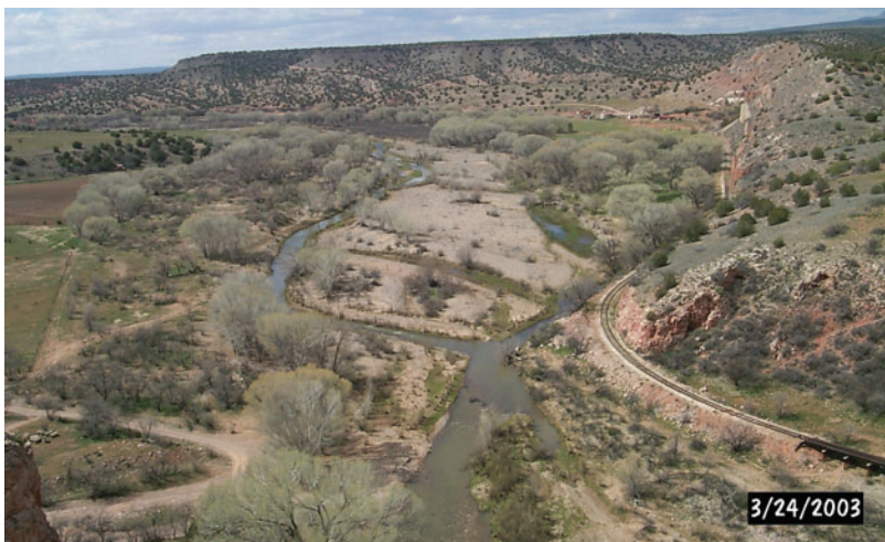
Figure 2.42 —A 2003 repeat photograph of the 1925 photograph (fig 2.41) of the Perkinsville area looking northwest along the Santa Fe Railroad (Verde River Railroad) toward the Station (light colored buildings in the upper right quadrant). Cottonwoods have established along old channels. This river segment of private land still remains a refuge for native minnows. (Photo by Alvin L. Medina.)
