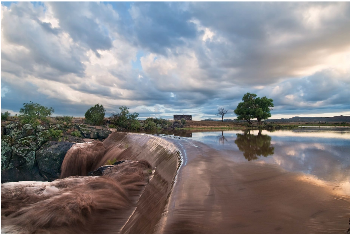
Fig 11. Sullivan Dam in flood at river mile 0. Gary Beverly Photo
